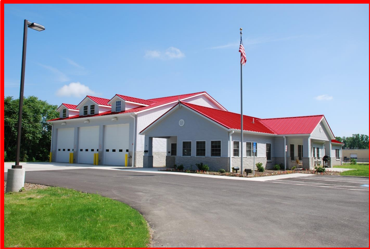
Barberton Fire Station 2, 93 E. State Street
