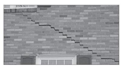
This home in Sugarcreek, Tuscarawas County, was damaged by the collapse of an underground mine. July 9, 2009.
